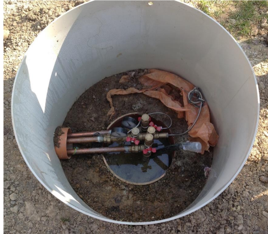
Geothermal borehole detail
