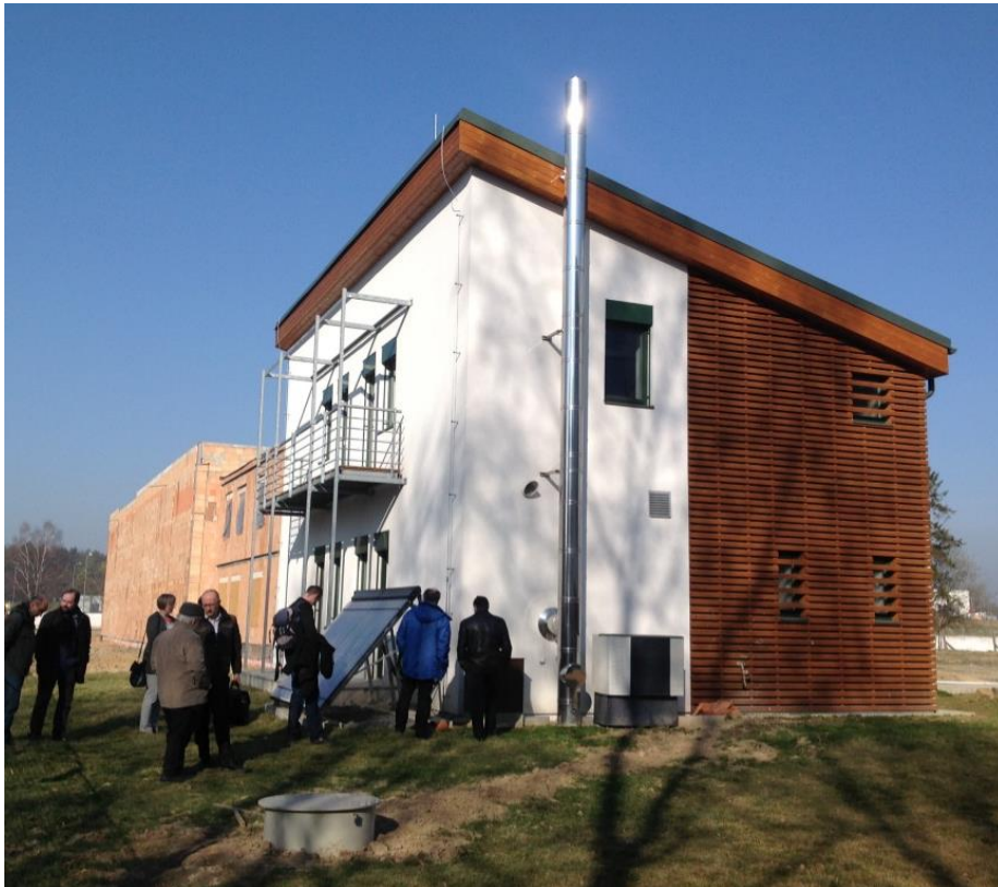
Passive house with geothermal borehole (in front)
